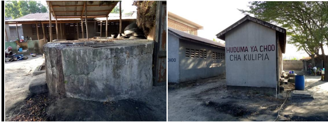
Figure 3: Some of the structures at the project site
